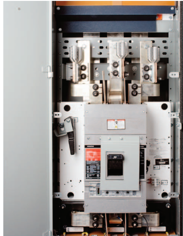
Main Circuit Breaker (MCB) Top Feed
