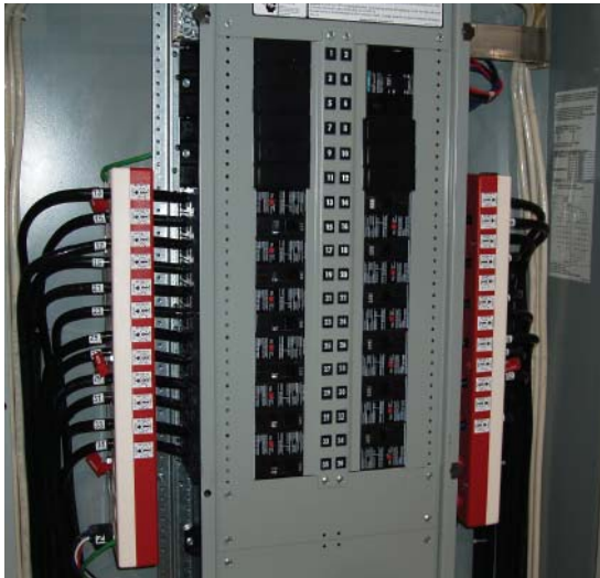
P2 panels with MP636-INC internal CT units installed in gutters.
