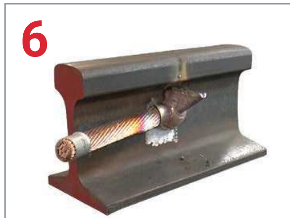
After reaction, open the mold and remove the expended steel cup – no special disposal required.
